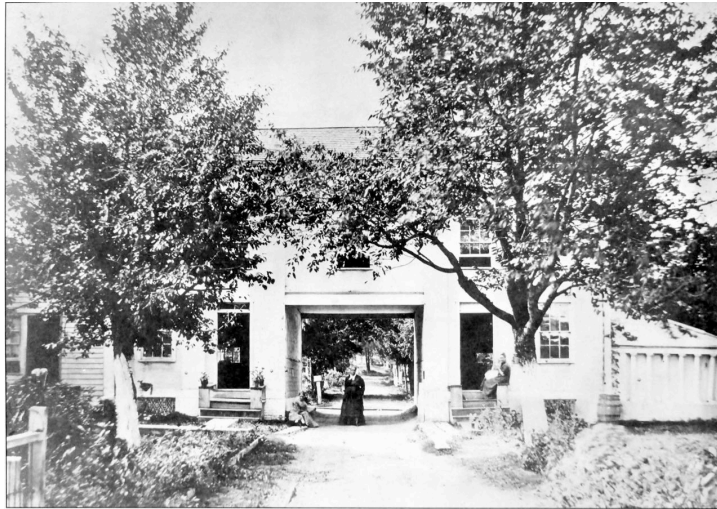
Lewisburg Cemetery Gatehouse built 1849. Union County Historical Society photo
