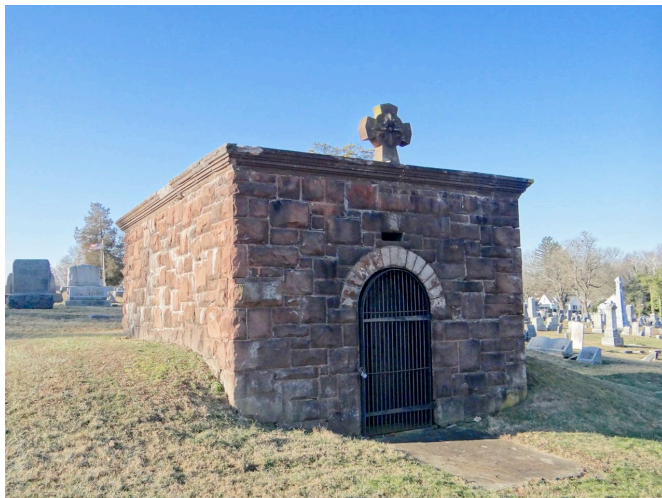
Lewisburg Cemetery vault built 1899. Greaves photo
